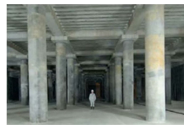
Sanno No. 2 stormwater detention chamber
