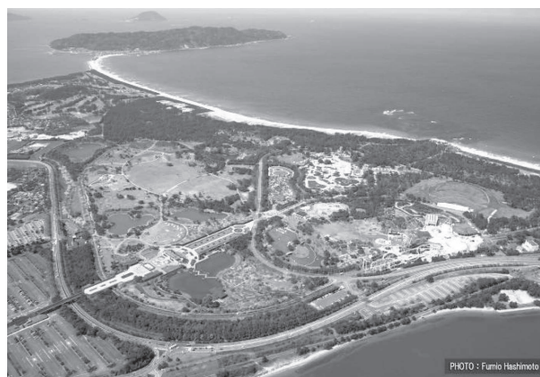
Photo 2 Uminonakamichi Seaside Park and Shikanoshima Island (Courtesy: Fukuoka City 9) )
